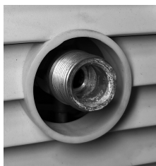
← High Pressure Hose Connection
